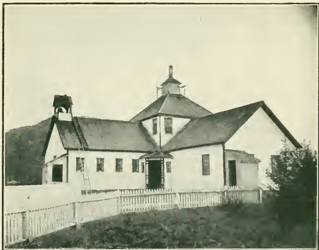
EDUCATIONAL BUILDING AT METLAKAHTLA
